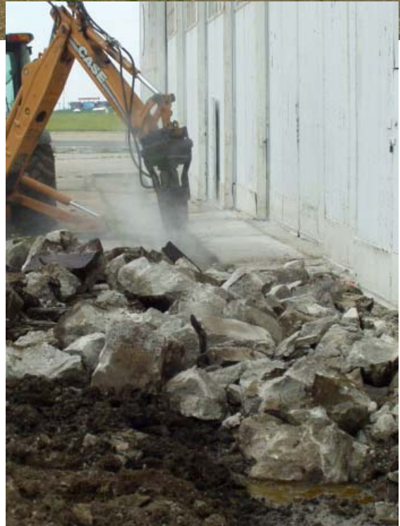
(Top) A section of existing concrete (Above) Concrete at the center front of the hangar was 15 to 18 inches thick. (Left) The new trench storm drain.
