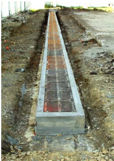
(Top) A section of existing concrete (Above) Concrete at the center front of the hangar was 15 to 18 inches thick. (Left) The new trench storm drain.
